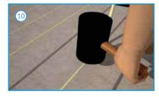
Start to push the pipe into the Retro-Fit Screed Board ensuring the pipe is fixed beneath the surface of the board (preferably using a rubber mallet to ensure a good fixing).
