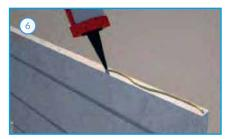
Work your way back up the room, staggering the panels as you go. Ensure you apply the 3mm bead of Retro-Fit Screed Board glue to all edges.
