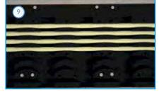
Start to roll the pipe into the End Support, utilis ing the self-retaining pipe clips, and continue to push the pipework into the connecting pipe runs until you reach the other end of the room.
