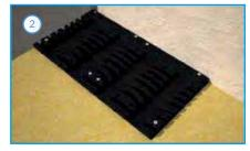
Start by laying the first two End Supports into the corner of the room and fix to the wood floor using the available screw holes.
