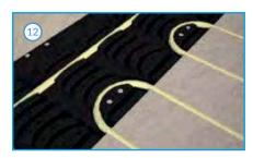
Continue to lay the pipe along the room until you reach the opposite end by walking the pipe into the groove as you go. Once you reach the end of the room, use the End Support to return the pipe back towards the other end.
