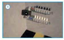
Start by fixing the manifold to the wall, about 500mm from the floor to the top of the flow meters. Connect the first circuit to the manifold with the euro cone adaptors
