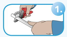
Cut the pipe square using a guillotine cutter.
