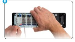
Connect the thermoelectric actuators wires.
