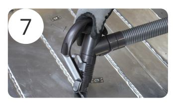
Sweep the panels to ensure they are free from debris, paying particular attention to the grooves. Then make sure no other trades are in the room when laying pipe to stop contamination.
