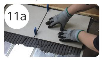
Fix the tiles using Mapei Keraquick S1 incorporating Mapei Latex Plus additive
