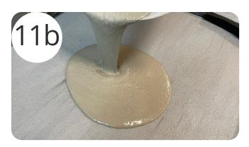
Using Mapei Ultraplan Renovation Screed 3240, mix up and pour to the depths shown in the table below. Once fully cured, tiles can be bonded using Mapei Keraquick S1 tile adhesive \*
