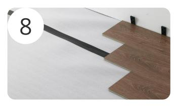
Before laying a laminate or engineered floor, we recommend using an underlay to help spread the heat and reduce system noise. The underlay should be approved for use with underfloor heating.
