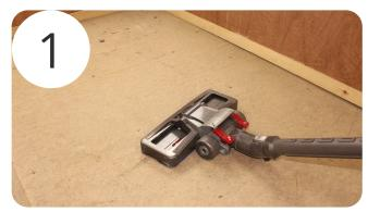
Ensure the subfloor is dry, clean and free from debris. Any holes/ uneven areas should be levelled using a suitable levelling compound.
