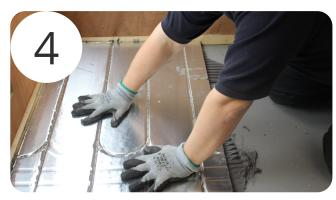
Lay the boards on the adhesive. As you go across the floor ensure full compression of the adhesive bed to the panel, also check as you go that the panels remain level.
