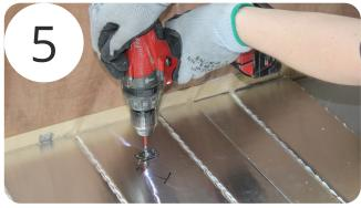
If fitting to a timber subfloor, we recommend large flange head fixing screws every 300mm across the entire board as well.
