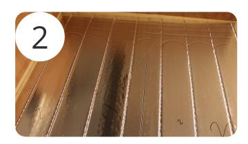
Using your supplied UFH drawing, ensure the panels are laid in the directions shown and do any cuts required to make the boards fit.
