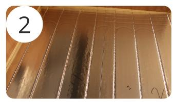
Using your supplied UFH drawing, ensure the panels are laid (loosely) in the direction shown and complete any cuts required to make the boards up.
