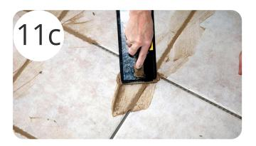
Once cured tiles can be grouted using Mapei Ultracolor Plus. Allow to fully cure before walking on the surface.
