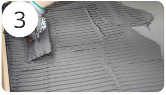
Apply Mapei Keraquick S1 adhesive to the subfloor using a notched trowel to give a minimum 3mm adhesive bed. (The adhesive bed depth may need to increase if the substrate is not sufficiently level). Levelling compound may be required if areas are any deeper than 2-3mm. This needs to be fully cured before continuing.
