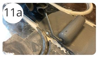
If using a levelling compound, prime the board with Mapei Eco Prim Grip using a brush or roller and ensure you cover the entire board and pipework. Leave to dry for a minimum of 60 minutes
