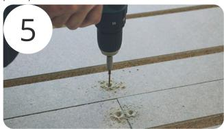
Fortis Timber Panels should then be screwed to the joist or batten with a countersunk screw (50–75mm in length). The screws need to be placed in the centre and edges of the board 350–450mm apart.
