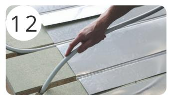
Thread the flow pipe through the board and run enough off your coil to get back to the manifold and we highly recommend connecting this to the flow manifold and stapling back to the wall.
