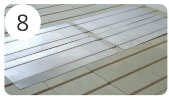
Install the heat transfer plates by pressing them to the Fortis Timber system. Please ensure a minimum of 10mm gap between plates. There is no requirement to bond the heat transfer plates to the base.
