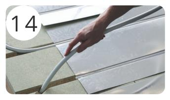
Now cut your coil allowing enough to get back to your manifold. Pass the remainder of the loop back through the return hole you made earlier and back to the manifold to make the final connection.
