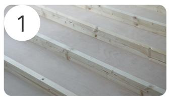
Install Fortis Timber boards so they run against the direction of the joists or battens. The joist or batten centres must be no greater than 600mm apart (minimum of 3-floor support areas per board). Where the joists are further apart, additional support should be installed and spaced accordingly. For further information, call our technical team on 01245 850799 or consult a structural engineer.
