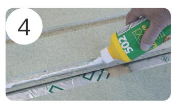
Always glue the boards at the base to avoid creaking and to each other at the tongue & groove on all four sides. Use an appropriate PVA (water-resistant) wood glue. Carefully apply the glue ensuring a continuous seam of adhesive along the board's entire length. Note: excessive use of glue might lead to gaps between the boards after drying. Before installing boards, check that the joists are even and level. Ensure panels that finish near walls and pillars are correctly supported.
