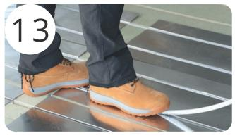
Install the heating pipes into the grooves of the heat transfer plates. Make sure that the pipe is fully pressed into the groove. To ensure the pipe sits down into the groove press in using your foot (best to use a soft bottom shoe and please ensure no sharp objects are embedded in the bottom of your shoe).
