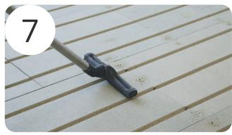
Before installing the Fortis Timber Heat Emission Plate, the floor and the pipe grooves should be cleaned of sawdust and other debris, to ensure no damage to the pipe system
