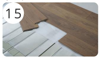
Both engineered, and laminate flooring can be installed directly on the heat transfer plates. We recommend using a low TOG underlay that is approved for underfloor heating. Use a minimum of 8mm engineered wood or laminate.
