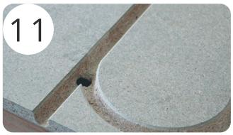
Before laying the pipe in the room drill a minimum 20mm hole in the groove closest to the room entry, this where the pipe will feed in from and do the same for the return.
