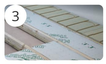
Start installation in the furthest room from the manifold to enable easy installation of the feed pipes between the rooms and the manifold.
