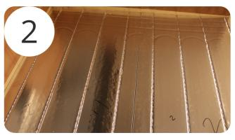
Using your supplied UFH drawing, ensure the panels are laid in the directions shown and do any cuts required to make the boards fit.
