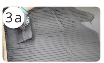
Apply Mapei Keraquick S1 adhesive to the subfloor using a notched trowel to give a minimum 3mm adhesive bed. (The adhesive bed depth may need to increase if the substrate is not sufficiently level). Levelling compound may be required if areas are any deeper than 2-3mm. The Adhesive needs to be fully cured before continuing.
