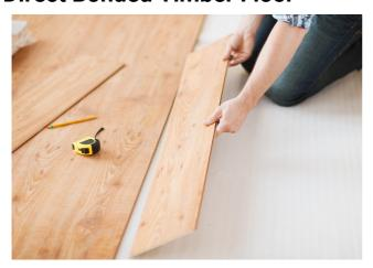
First, follow the preparation and laying steps from page 3, "Installation for Bonded System" (steps 1-10). Check with your wood floor supplier with suitability to directly bond the wood flooring to the UFH system. If they need a separation layer, follow the instructions on page 4, "laying with levelling compound".
