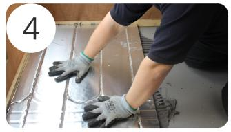
Lay the boards onto the adhesive and press down to the bed onto the adhesive. As you go across the floor, ensure full compression of the panel to the adhesive bed. Also, check as you go that the panels remain level and the grooves align.
