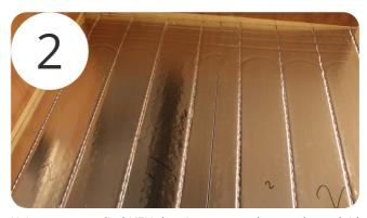
Using your supplied UFH drawing, ensure the panels are laid (loosely) in the direction shown and complete any cuts required to make the boards up.
