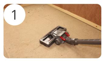
Ensure the subfloor is dry, clean and free from debris. Any holes/ uneven areas should be levelled using a suitable levelling compound.
