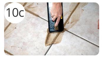
Once cured, tiles can be grouted using Mapei Ultracolor Plus. Allow the tiles to fully cure before walking on the surface. All movement joints can be filled with Mapei Mapesil AC (for ceramic and porcelain tiles) or Mapei Mapesil LM (for natural stone tiles). Allow the tiled area to cure for a minimum of 10 days before turning the heating system on and heat up as per the guidance in the main UFH installation guide.
