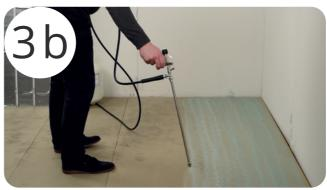
As an alternative, you can use a spray impact adhesive. If you decide to use a spray adhesive, ensure it is compatible with the subfloor and polystyrene insulation. A suitable product is 3M™ Hi-Temperature Polystyrene adhesive 78HT. But please ensure compatibility.
