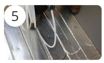
Referring to the UFH drawing, pick the pipework for each room that you intend to use. Using either a decoiler or by hand lay the pipework into the pipe grooves, ensuring it is pressed into the grooves.
