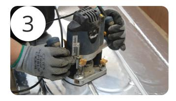
If you need to alter the panels, we recommend using a knife or a router to channel a new route. Ideal for feeds or avoiding fixed furniture.
