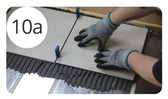
Fix the tiles using Mapei Keraquick S1 incorporating Mapei Latex Plus additive. Ensure that every pipe channel and void surrounding the pipe is fully encapsulated and covered with tile adhesive. Use a notched trowel to ensure good adhesion to the surface and tile.
