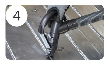
Sweep the panels to ensure they are free from debris paying particular attention to the grooves. Then make sure no other trades are in the room when laying pipe to stop contamination.
