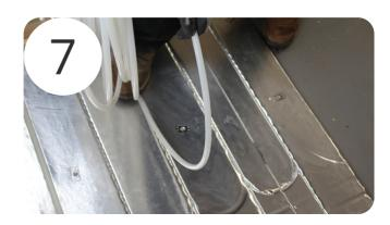
Referring to the UFH drawing, pick the pipework for each room you intend to use. Then using either a decoiler, or by hand, lay the pipework into the pipe grooves.
