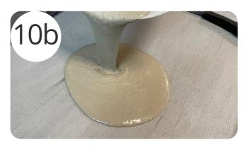
Using Mapei Ultraplan Renovation Screed 3240, mix up and pour to the depths shown in the table on Page 5. Once fully cured, tiles can be bonded using Mapei Keraquick S1 tile
