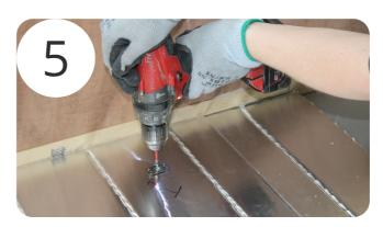
If fitting to a timber subfloor, we recommend large flange head fixing screws every 300mm across the entire board as well. Allow the adhesive to cure for a minimum of 3 hours (depending on temperature) but ideally overnight to ensure the adhesive is fully cured.
