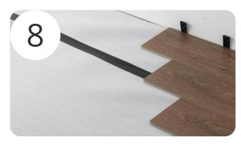
Before laying a laminate or engineered floor, we recommend using an underlay to help spread the heat and reduce system noise. The underlay has to be approved for use with underfloor heating systems.
